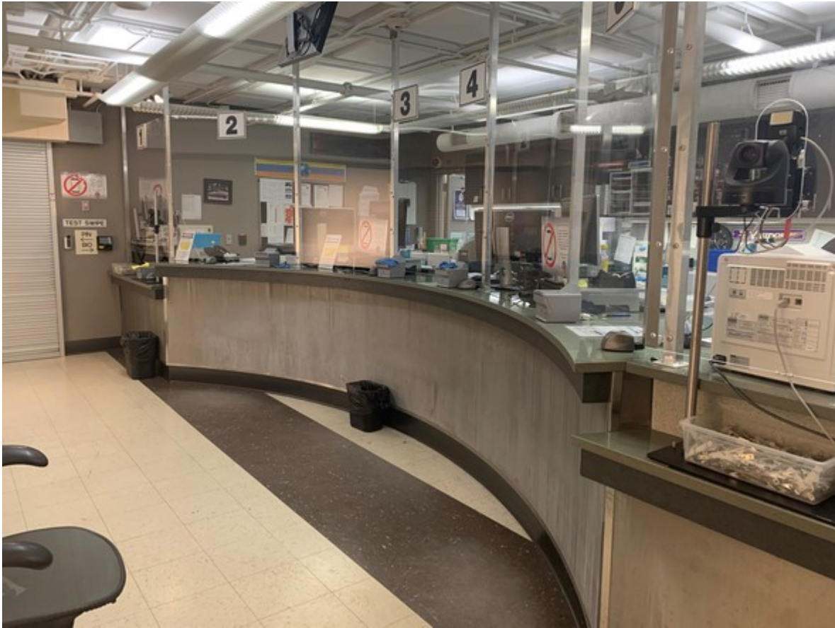
The new Plexiglas installed at the Badging Office's service counter.
