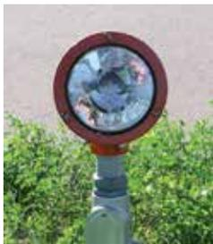
REILs consist of two synchronized white flashing lights, one on each side of the runway threshold, which provide rapid and positive identification of the approach end of a particular runway. Runways 30R and 17 are the only runways with this type of lighting at MSP.
