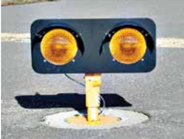
Runway Guard Lights (RGLs) are designed to facilitate taxiing during low visibility operations. These lights provide a distinctive warning to aircraft and vehicles that they are approaching a runway holding position, these lights do not indicate whether a runway is open or closed. Each elevated runway guard light fixture consists of two flashing unidirectional yellow lights. These are located at all taxiway feeder entrances to Runways at MSP.
