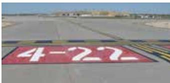
These signs have a red background with a white inscription and supplement the signs located at a runway holding position. At MSP, there are a set of two surface painted holding position signs at each taxiway feeder that intersects a runway.
