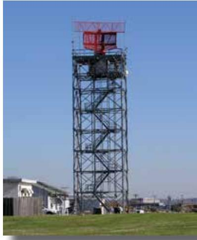
This radar is used by the air traffic control tower and provides the position of the aircraft in terms of azimuth and range data. It does not provide elevation data and is designed for range coverage up to 60 nautical miles.
