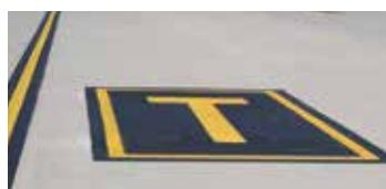
These signs have a black background with a yellow inscription and are used when it is not possible to provide a location sign along the edge of the taxiway or when it is necessary to supplement such signs. These signs are located on the right side of the taxiway centerline.
