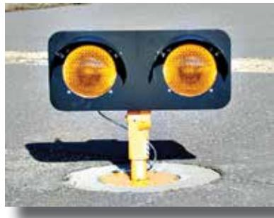
Runway Guard Lights (RGLs) are designed to facilitate taxiing during low visibility operations. These lights provide a distinctive warning to aircraft and vehicles that they are approaching a runway holding position, these lights do not indicate whether a runway is open or closed. Each elevated runway guard light fixture consists of two flashing unidirectional yellow lights. These are located at all taxiway feeder entrances to Runways at MSP.
