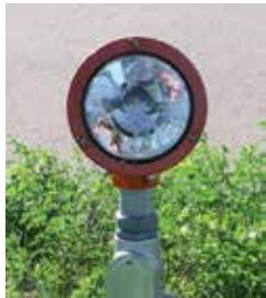
REILs consist of two synchronized white flashing lights, one on each side of the runway threshold, which provide rapid and positive identification of the approach end of a particular runway. Runways 30R and 17 are the only runways with this type of lighting at MSP.
