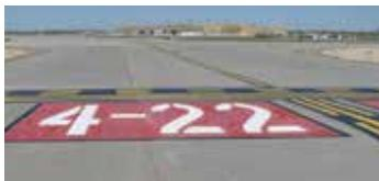
These signs have a red background with a white inscription and supplement the signs located at a runway holding position. At MSP, there are a set of two surface painted holding position signs at each taxiway feeder that intersects a runway.
