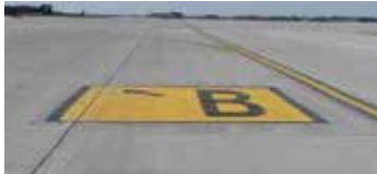
These signs have a yellow background with a black inscription, and are used when it is not possible to provide a taxiway direction sign along the edge of a taxiway at an intersection, or when necessary to supplement such signs. These signs are located adjacent to the taxiway centerline, with signs indicating turns to the left on the left side of the centerline and signs indicating turns to the right on the right side of centerline.
