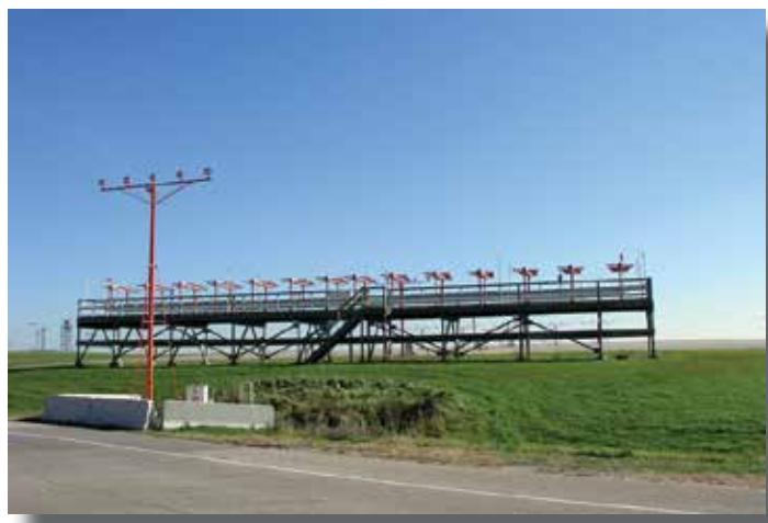
The localizer is another part of the ILS Navigation System and provides lateral guidance to aircraft on an approach to the runway. All runways at MSP have a localizer and it is typically located on the extended centerline of the runway, 1,000 feet beyond the departure end.
