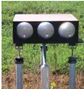
These lights consist of 4 lamp boxes and are normally located on the left side of the runway as viewed from the approach direction approximately 1,000 feet from the threshold. The PAPI's furnish the pilot with visual approach slope information to provide guidance for safe descent. This system is intended primarily for use during Visual Flight Rule (VFR) conditions or clear sky and good visibility conditions.
